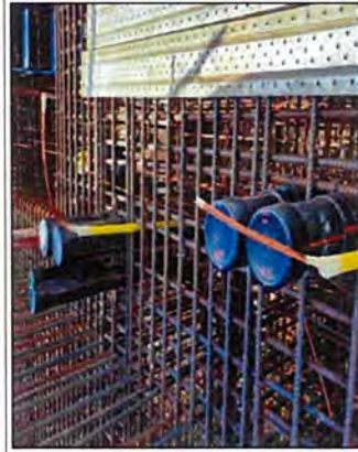
Grounding, riser and HDPE conduit installation
