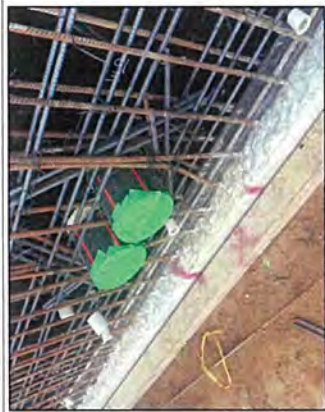
Grounding, riser and HDPE conduit installation
