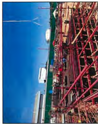
Rebar, formworks and embedded item installation for CT/G #71
